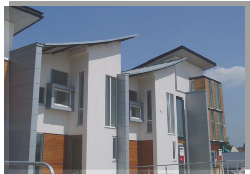
Client: New East Manchester Project: 550 mixed tenure homes Contract value: £60m
